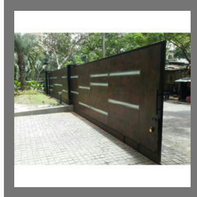
Motorized Sliding Gate
