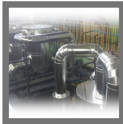
Hot Insulation Works And Services
