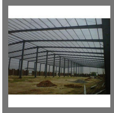
PEB Structural Shed
