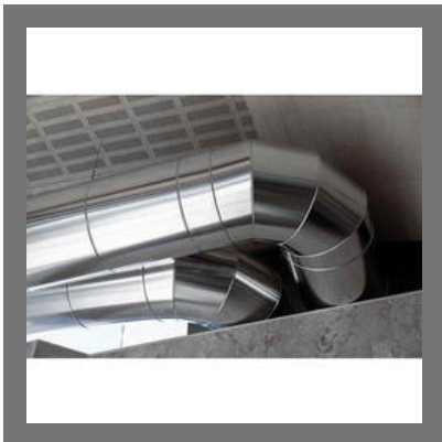
Stainless Air Conditioning Duct
